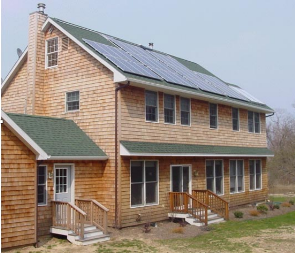
Fig 2.: ZEH home on Long Island, courtesy of Solar Strategies Development Corp.
