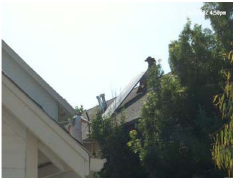
Figure-4 Installation of first 4' wide module. (Photo by Energy Ideas)
