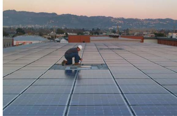
Photo-1 PowerGuard BIPV installation (Photo courtesy of PowerLight).
