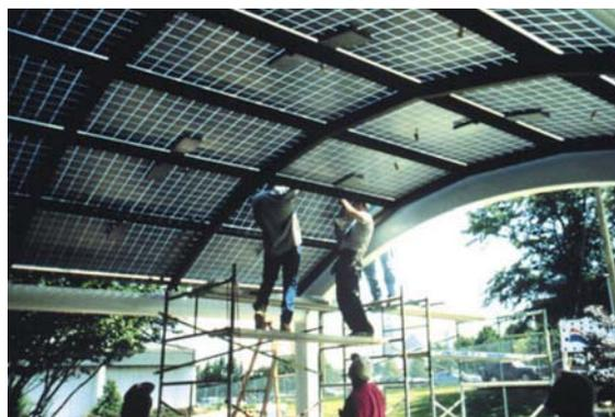
Photo 4. AC PV Modules (Photo Courtesy of NREL).
