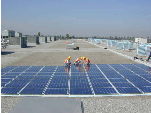
Photo 5. PowerLight Roof Installation (Photo Courtesy of PowerLight).
