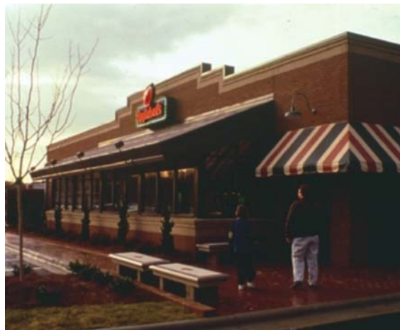
Photo 3. Architectural PV Awning, PV Below Sign (Photo Courtesy of NREL).
